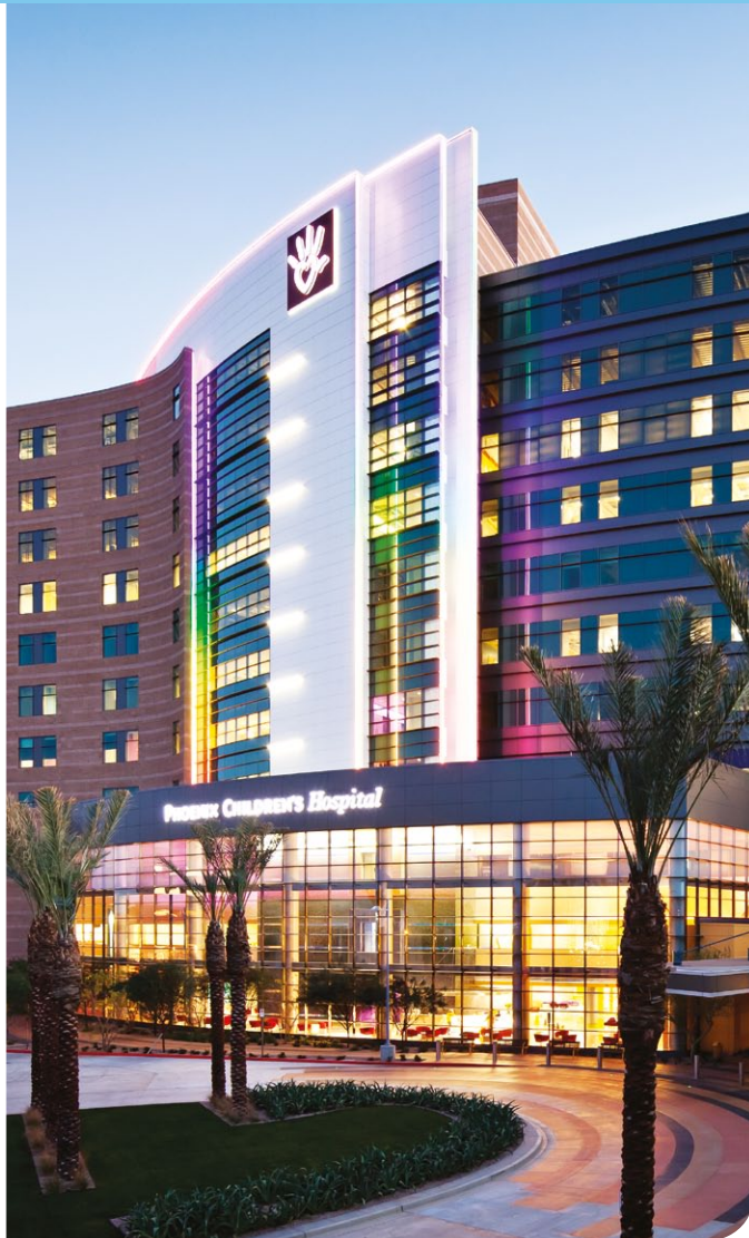
Phoenix Children's Hospital: The iColor Accent MX is used to enhanced 3-dimensional outlines of the building without disturbing light pollution affecting the interior.
